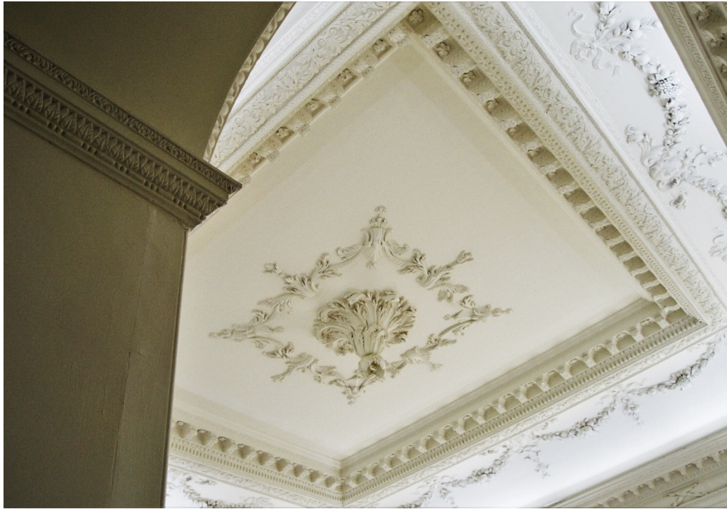
Figure 19 Staircase Hall Ceiling
