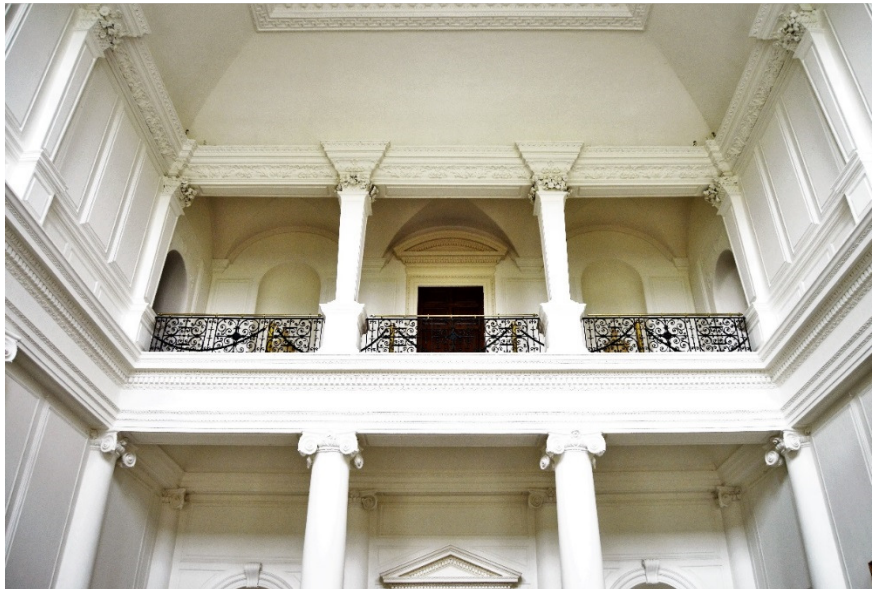
Figure 9 Entrance Hall Upper Level, 1st floor balcony
