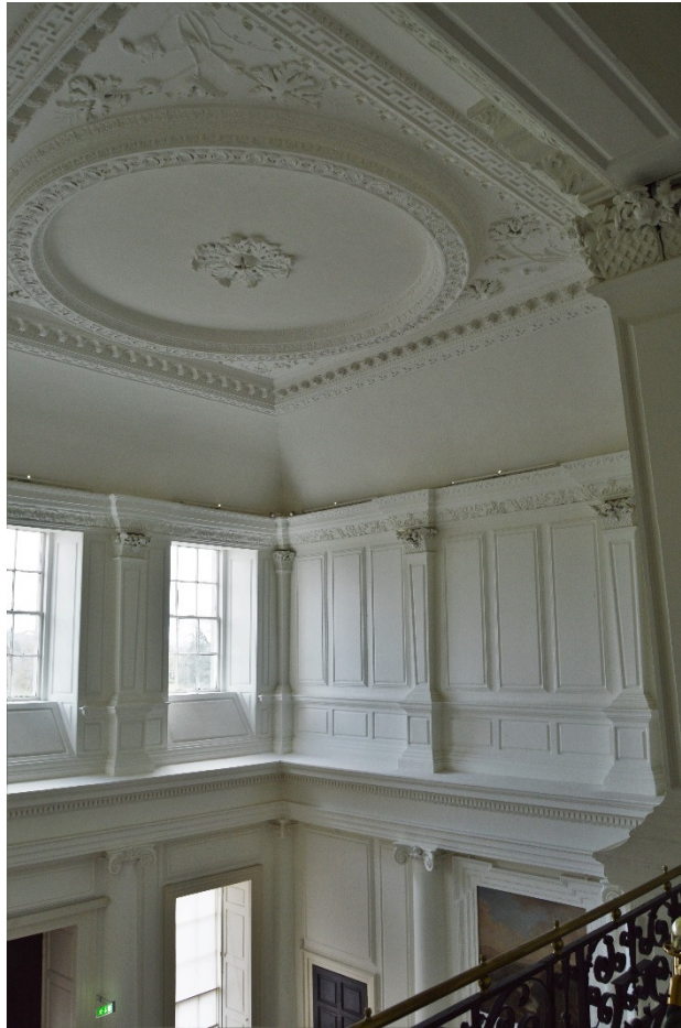
Figure 10 Entrance Hall Ceiling
